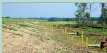
Completed Relief Wells and Berm at Buck Chute
