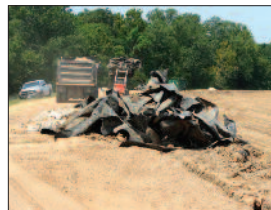
Removing Poly Sheetting
