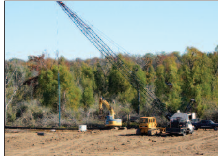
Installing Buck Chute Relief Wells
